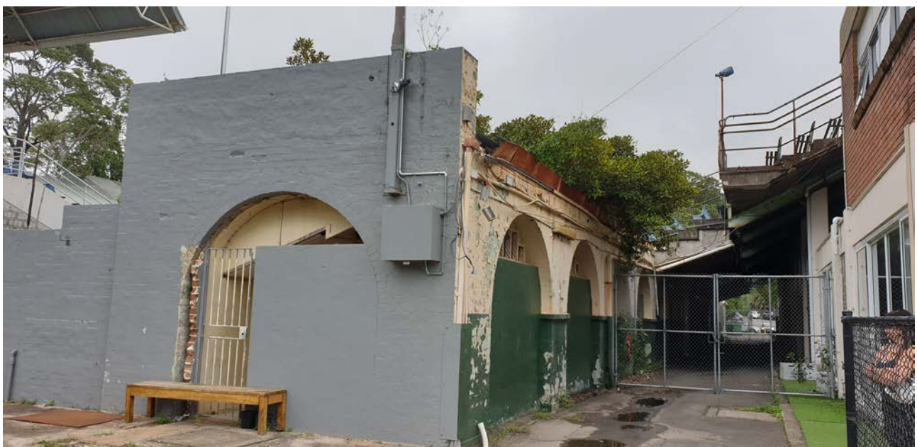
Figure 3: Remnants of the Northern Grandstand arches designed by Leslie Wilkinson, photo WMC 6 March 2020. The infill of the arches are reversible works that could be undertaken as part of the proposal.
